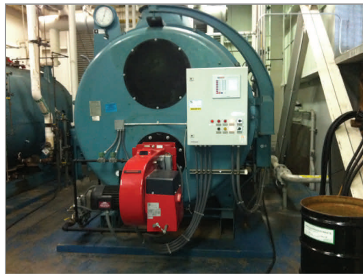
Burner and Control Upgrade
